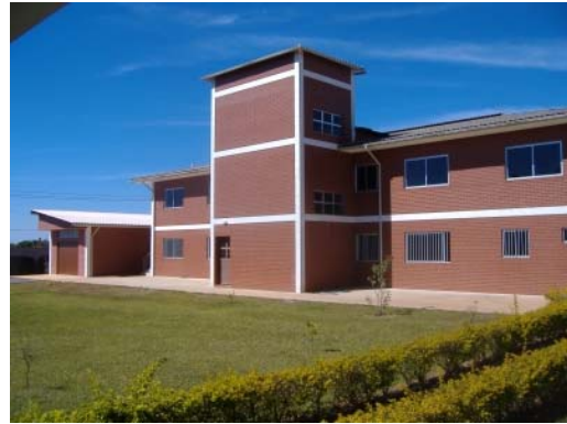
New Office and Storage Building
